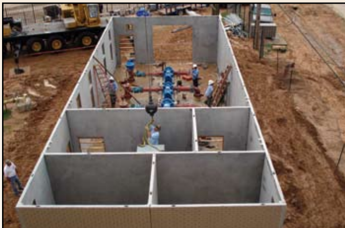
24' x 60' Building for the City of Humble, TX
